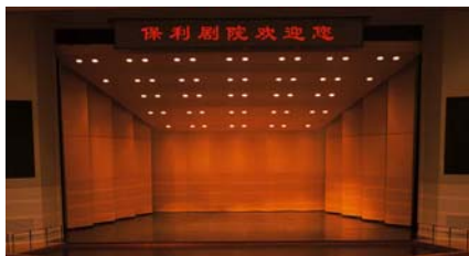
图 1 北京保利大剧院乐罩内景 Fig.1 Acoustic reflecting cover of Beijing Poly Theatre
