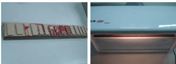
(a) Muffler (b) Installation of muffler
