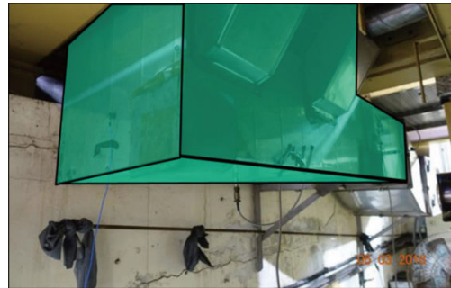
图 8 将通风管道理想化为三个虚拟平面 Fig.8 Dividing the ventilation duct into three virtual planes
